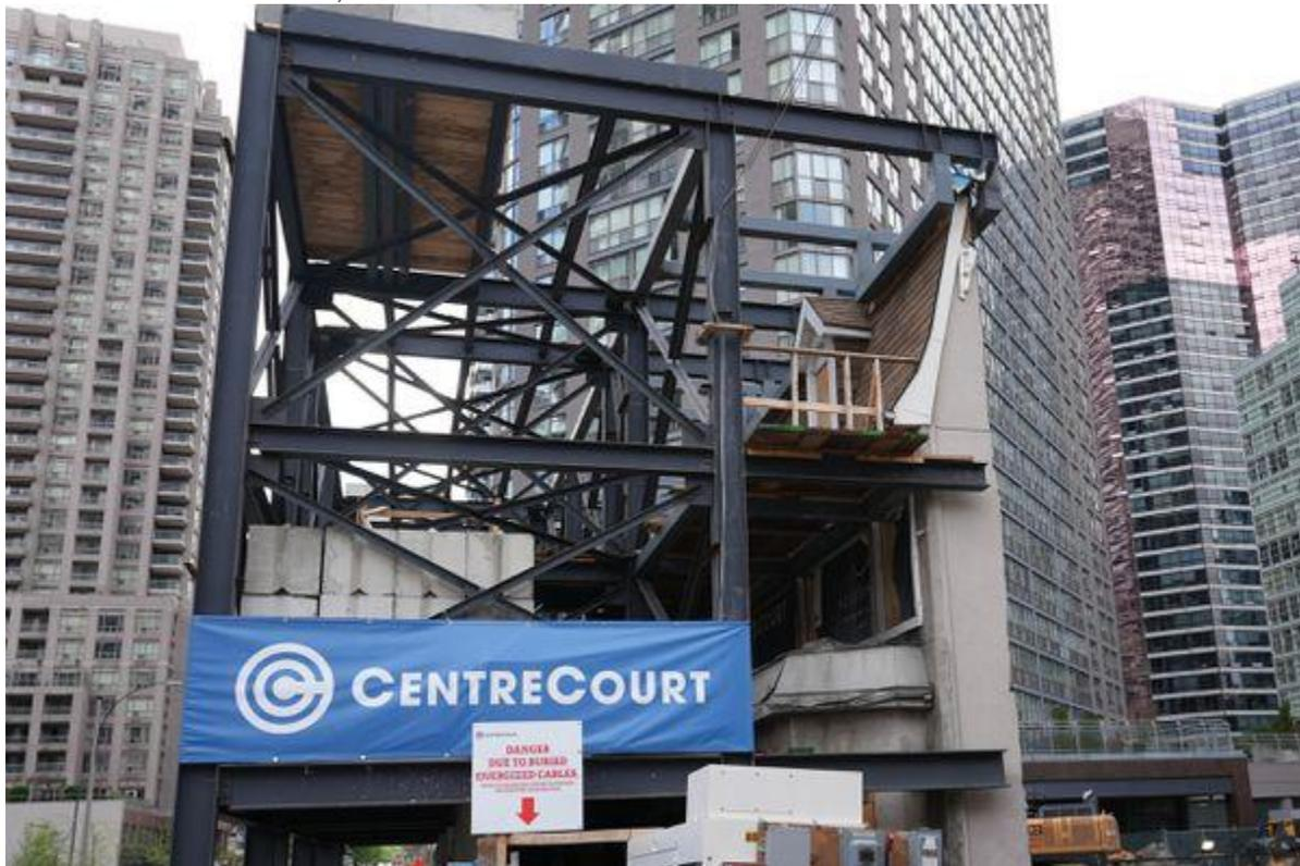
At Wellesley St. just west of Yonge St. in Toronto, we are able to see a steel retention frame holding up numbers 10 to 16. These two-and-a-half storey, bay windowed, Second Empire houses were built as speculative housing by Thomas Bryce of Bryce Brothers Construction in 1876. DYLAN AUTHORS
