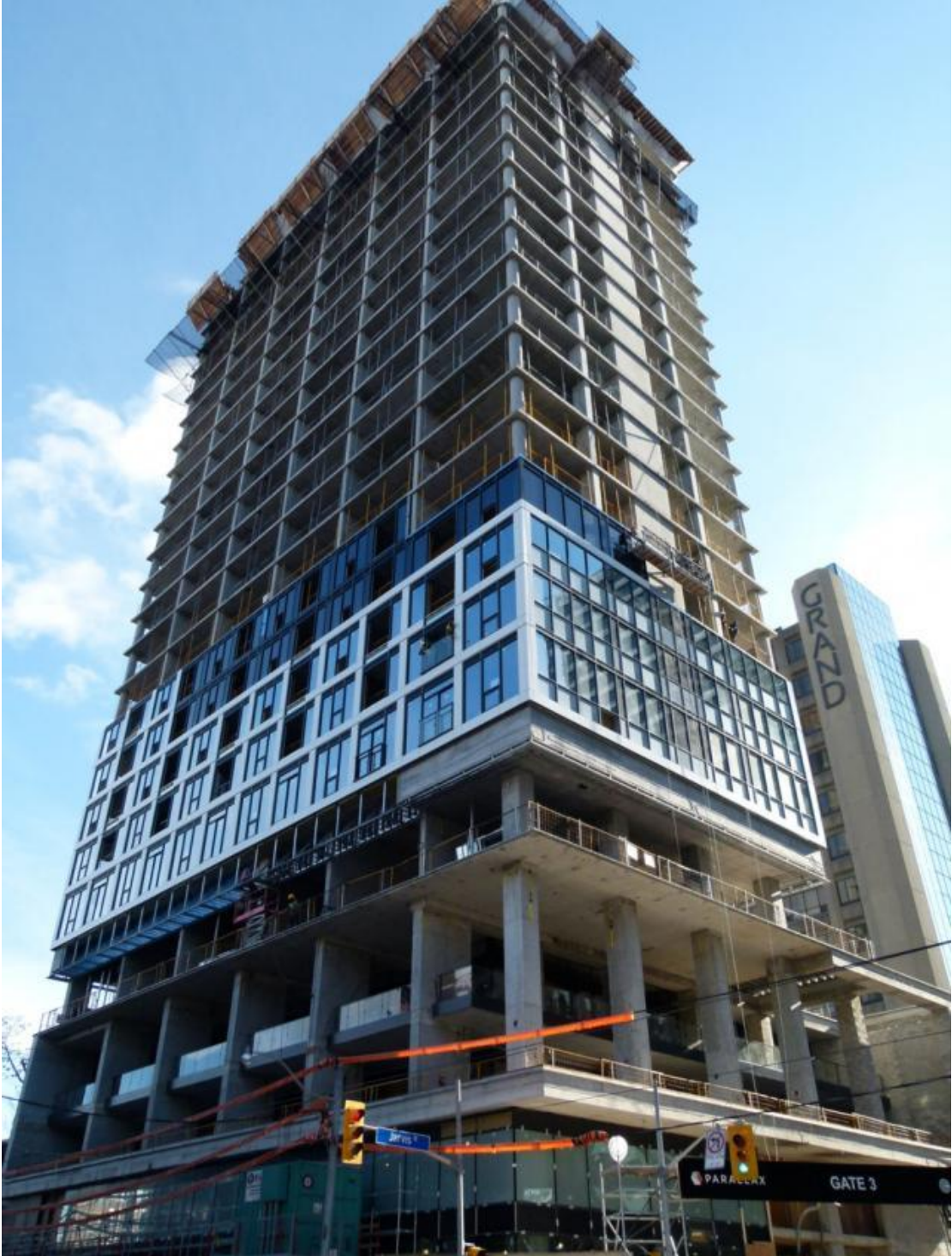
installation progressing for Grid Condos, image by Forum contributor skycandy
